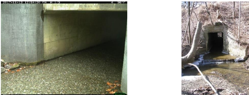
Figure 27. Examples of old box culverts with “sheetflow concrete” movement surface. Site 30-22 (West Townshend) and 15-76 (Cambridge, Marangelo and Farrelll 2016).
