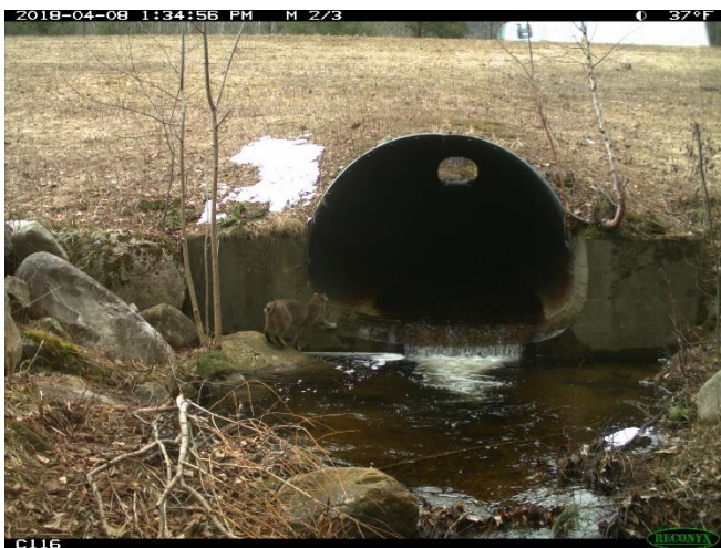
Bobcat at squash pipe 7-19-5, Sunderland
