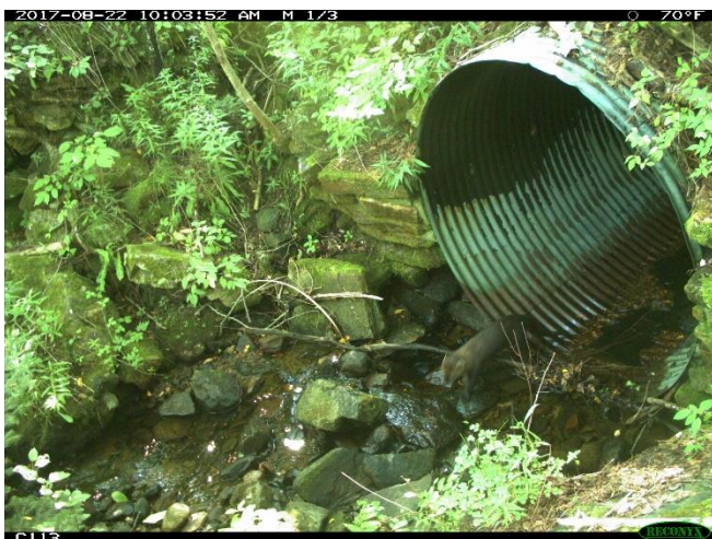
Fisher at pipe culvert 155-6, Mt Holly
