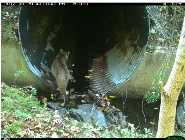
Bobcat at pipe culvert I91a, Sheffield
