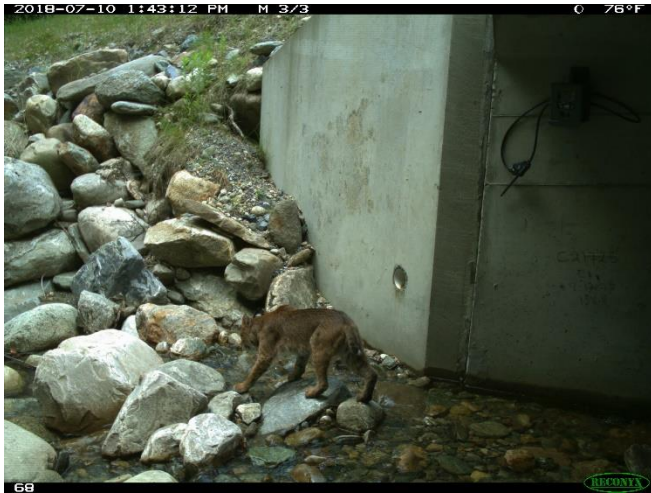
Bobcat at new precast box culvert 125-19, Ripton (only through-passage recorded for this site)
