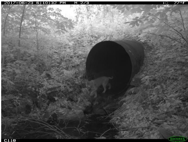
Bobcat at pipe culvert in Manchester (Site 7-19-5)
