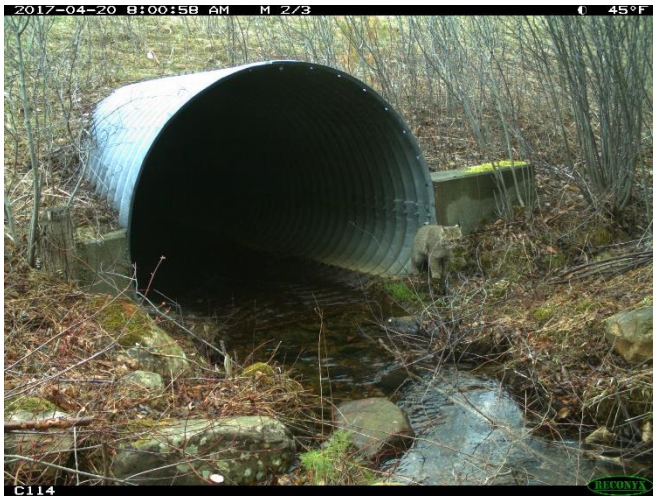
Bobcat at squash pipe in Sunderland, VT (Site 7-19-5)
