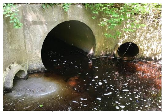
An example of a site stressed both by the culvert and stormwater (the two smaller pipes shown here are for stormwater discharge; note the large mound of sedimentation below the one on the left).
